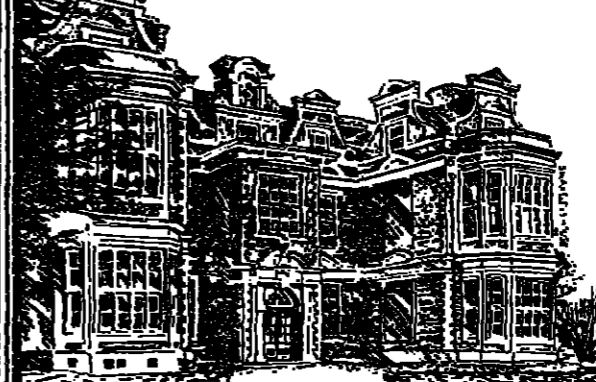
Stankov's House, Islington. This beautiful Jacobean Mansion was restored to its former glory by Try Construction Group.
